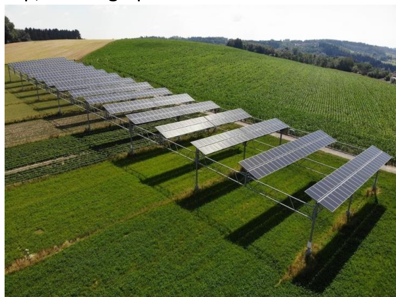
The agrivoltaic system in Heggelbach near Lake Constance in Germany. ("Agrophotovoltaics: Land use efficiency of up to 186 percent". Accessed July 2019 from https://www.pveurope.eu/News/Solar-Generator/Agrophotovoltaics-Land-use-efficiency-of-up-to-186-percent )
